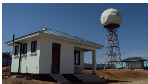
Figure 5: S- Band Meteorological Weather Radar Station
